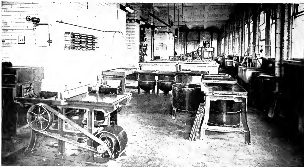
FIG. 27.—WAX SHAVER AND WAX HEATING, ELECTRIC HEATING DEPARTMENT.
